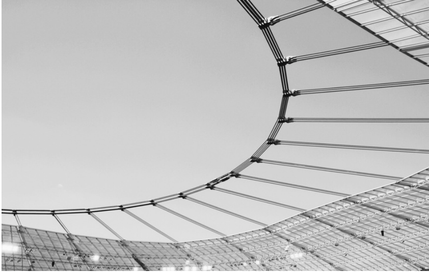
Detail vom Stadionsdach (innen)/detail of the stadium roof (inside)
